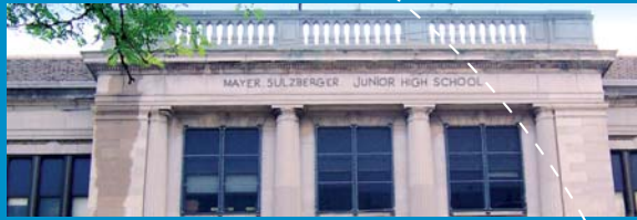
Facade Rehabilitation Mayer Sulzberger Middle School - Philadelphia, PA
